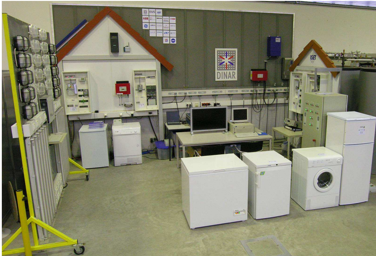
Test house of the IWES smart grid laboratory
