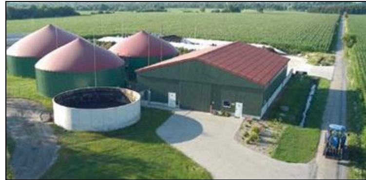
Biomass power plant / CHP
